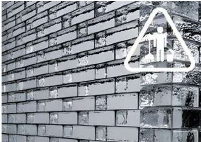
2.5 The glass wall can be scrubbed 24 hours after the completion of wall laying.
