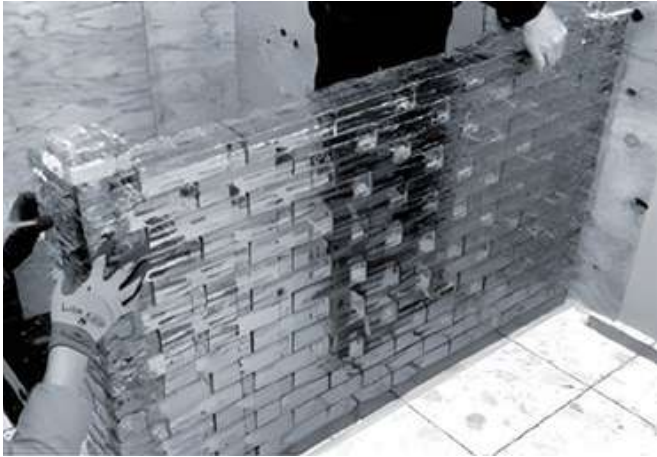
2.1 Level the ground, try placing the first layer of bricks, and stick them firmly after confirmation.
